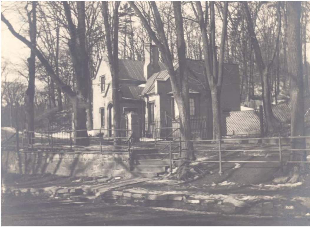
Figure 10. The gatekeepers lodge in a photograph from c.1910.
