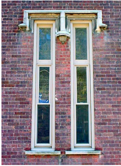
Figure 15. Stockbridge marble lintel, 2006.
