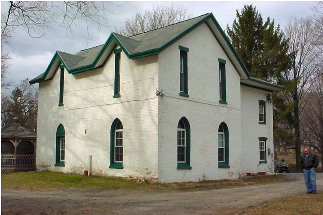
Figure 11. The gardener's cottage, 2006.
