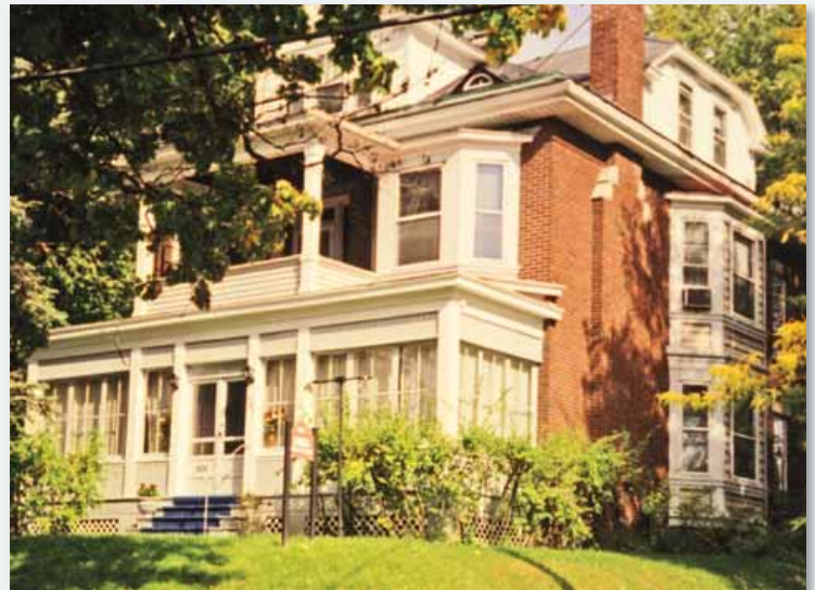
Begun in 1971, The Abba House of Prayer on Western Avenue welcomed laity, priests and religious for prayer. Following its closing several years ago, it will serve as a community house for RSCJ in the Albany area.
